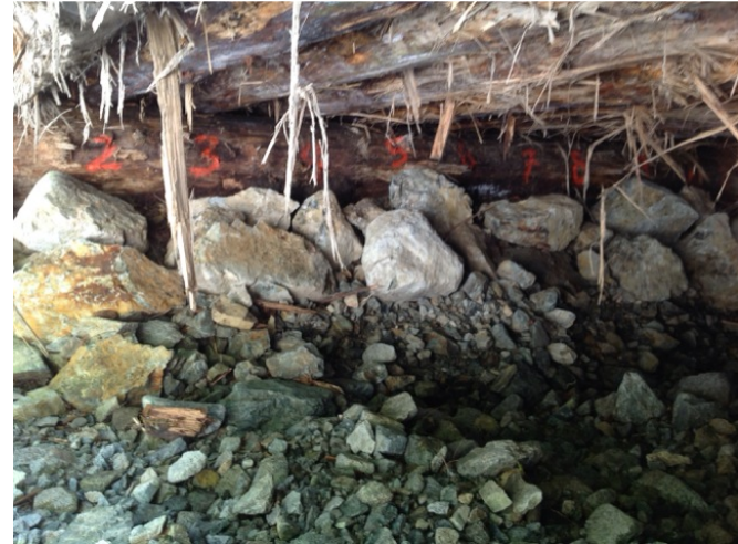
Left Bank Abutment when facing downstream
