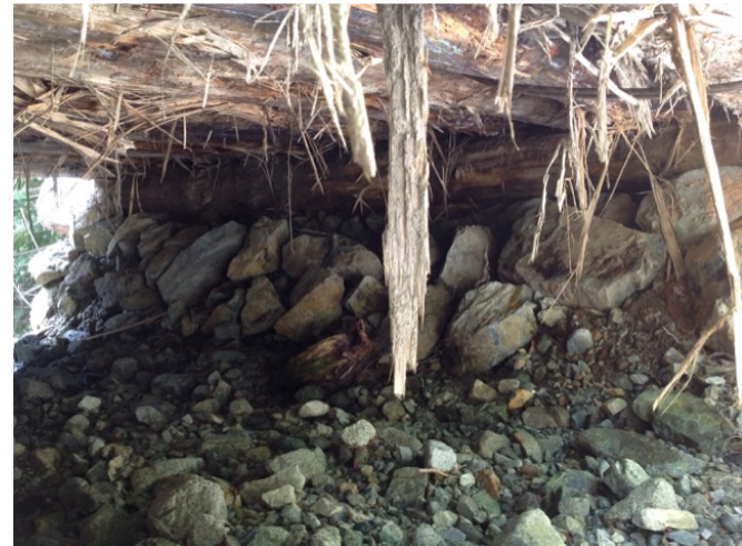
Right Bank Abutment when facing downstream
